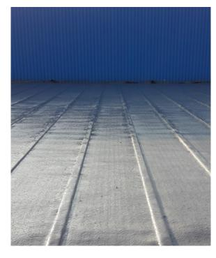
Depending on the quality, porosity, or nature of the substrate to be coated, or the type of product to be used, it may be necessary to apply, with a consumption of 0.02 to 0.09 lb/ft² (0.100 to 0.450 kg/m²), one of the following primers: NEXA PRIMER EPOX W or NEXA PRIMER PU 2K. Some waterproofing applications may require a vapor barrier, which can be created with NEXA PRIMER EPOX W (0.12–0.20 lb/ft² (0.6–1 kg/m²) depending on the substrate's porosity). (See www.nexacoatings.com)
