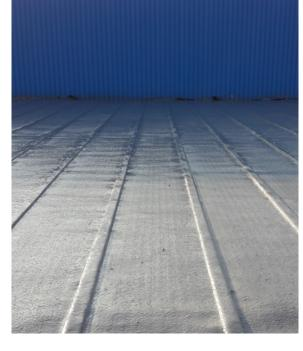
Depending on the quality, porosity, or nature of the substrate to be coated, or the type of product to be used, it may be necessary to apply, with a consumption of 0.02 to 0.09 lb/ft² (0.100 to 0.450 kg/m²), one of the following primers: NEXA PRIMER EPOX W or NEXA PRIMER PU 2K. Some waterproofing applications may require a vapor barrier, which can be created with NEXA PRIMER EPOX W (0.12–0.20 lb/ft² (0.6–1 kg/m²) depending on the substrate's porosity). (See www.nexacoatings.com)
